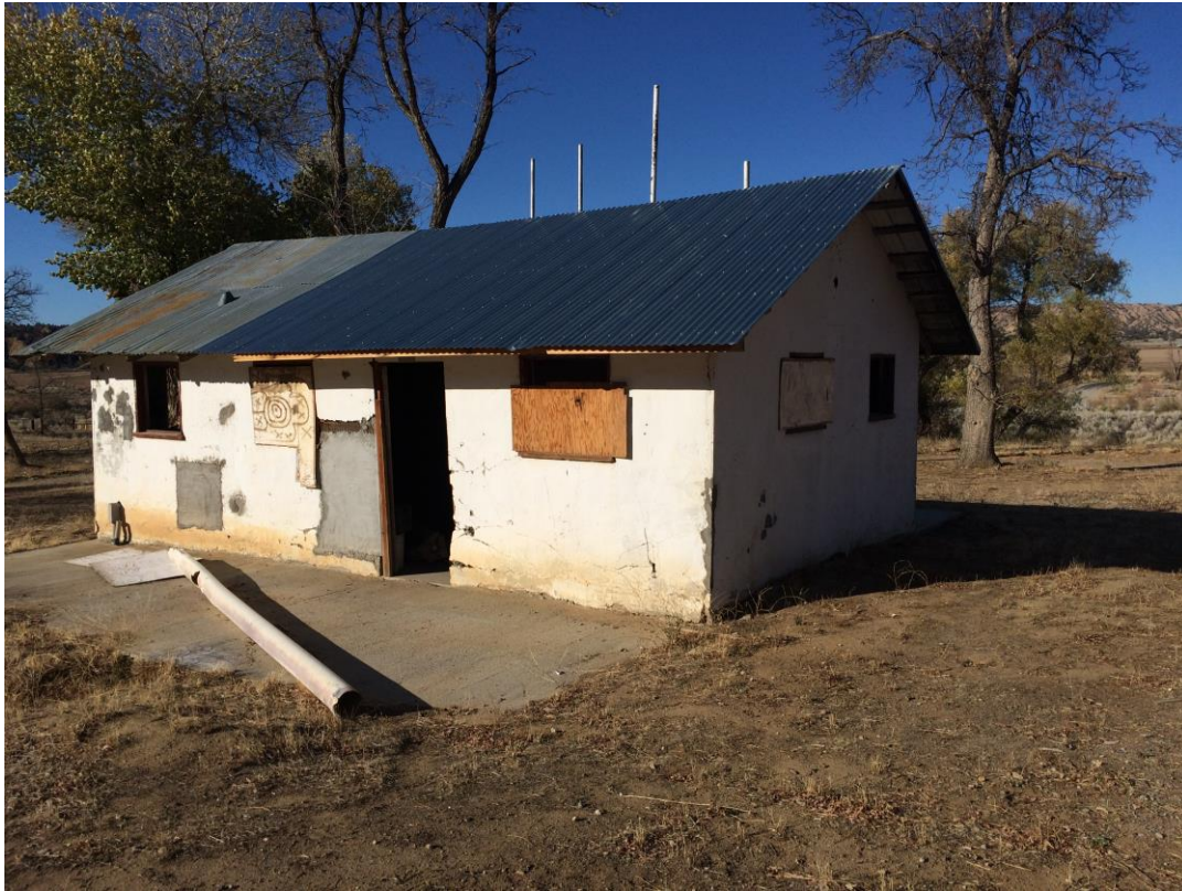
Figure 10. View of washroom constructed on the property in 1947, view looking northwest.
