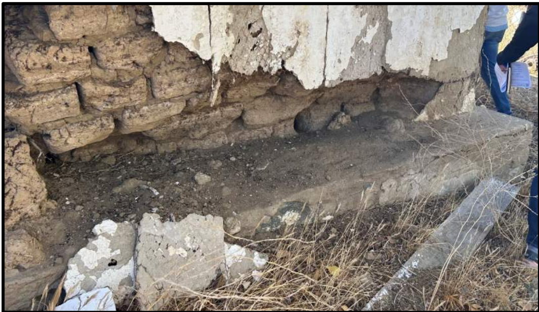
Underpinning Replacing Lower Portion of Adobe Wall
