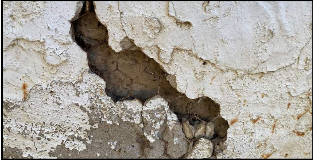
Parge Coat & Metal Lath Over Adobe
