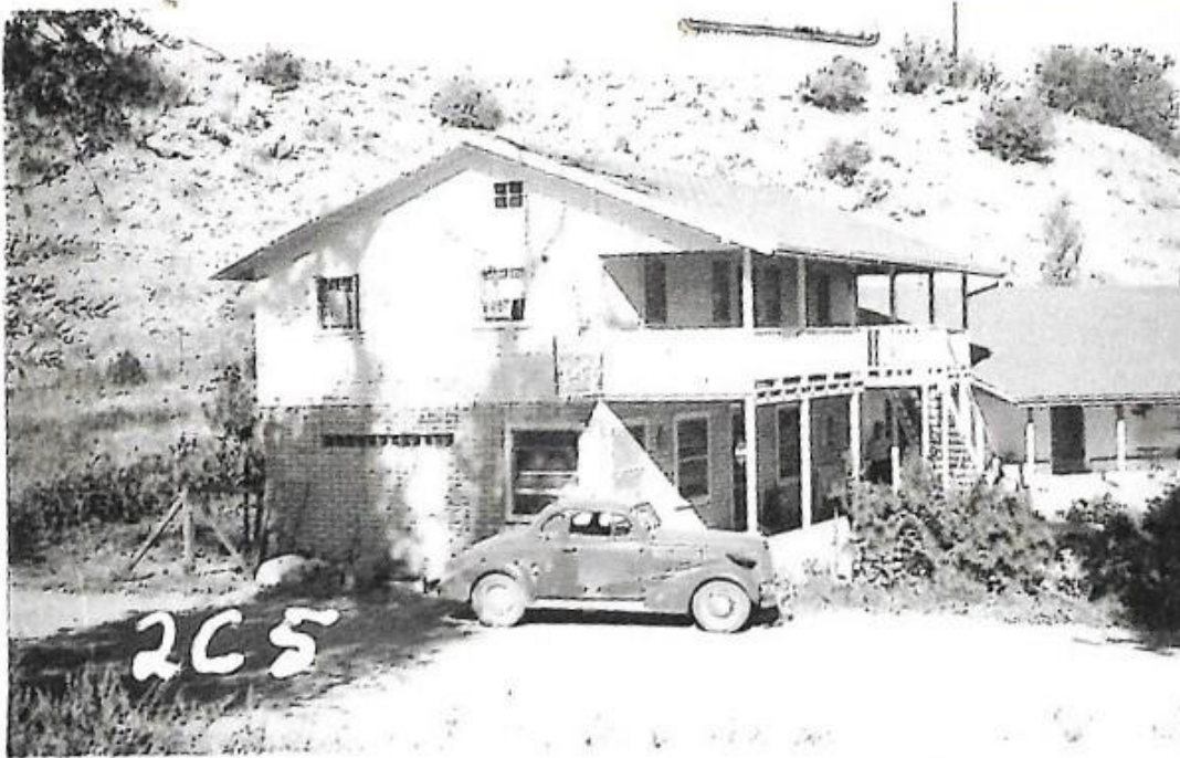
Figure 7. County Assessor Records showing adobe and addition in 1952.
