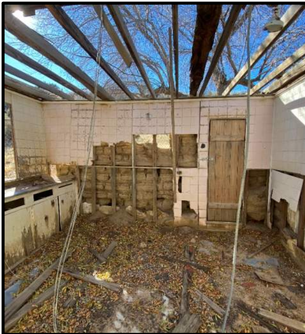
Remnants of Ceiling Framing at South End of Adobe (left) and Collapsed Roof at North End (right)
