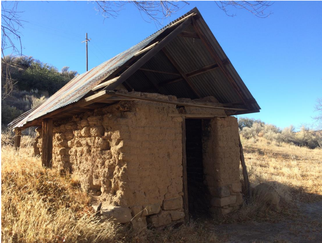
Figure 20. East façade of smokehouse, view to the northwest.
