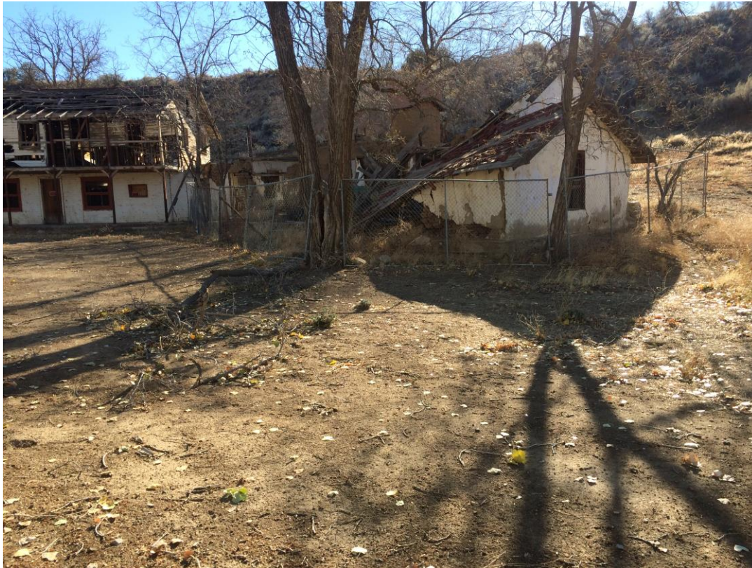
Figure 8. Overview of adobe and addition looking southwest.
