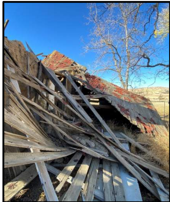
Remnants of Ceiling Framing at South End of Adobe (left) and Collapsed Roof at North End (right)
