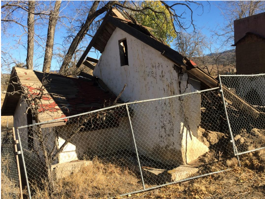
Figure 12. Detail of addition walls which are still standing, looking southeast.
