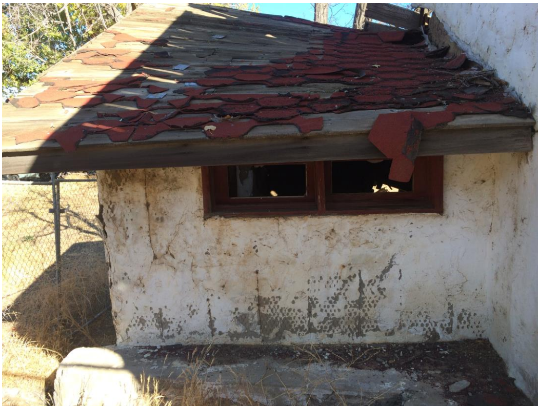
Figure 13. Detail of clerestory window on west façade of addition.
